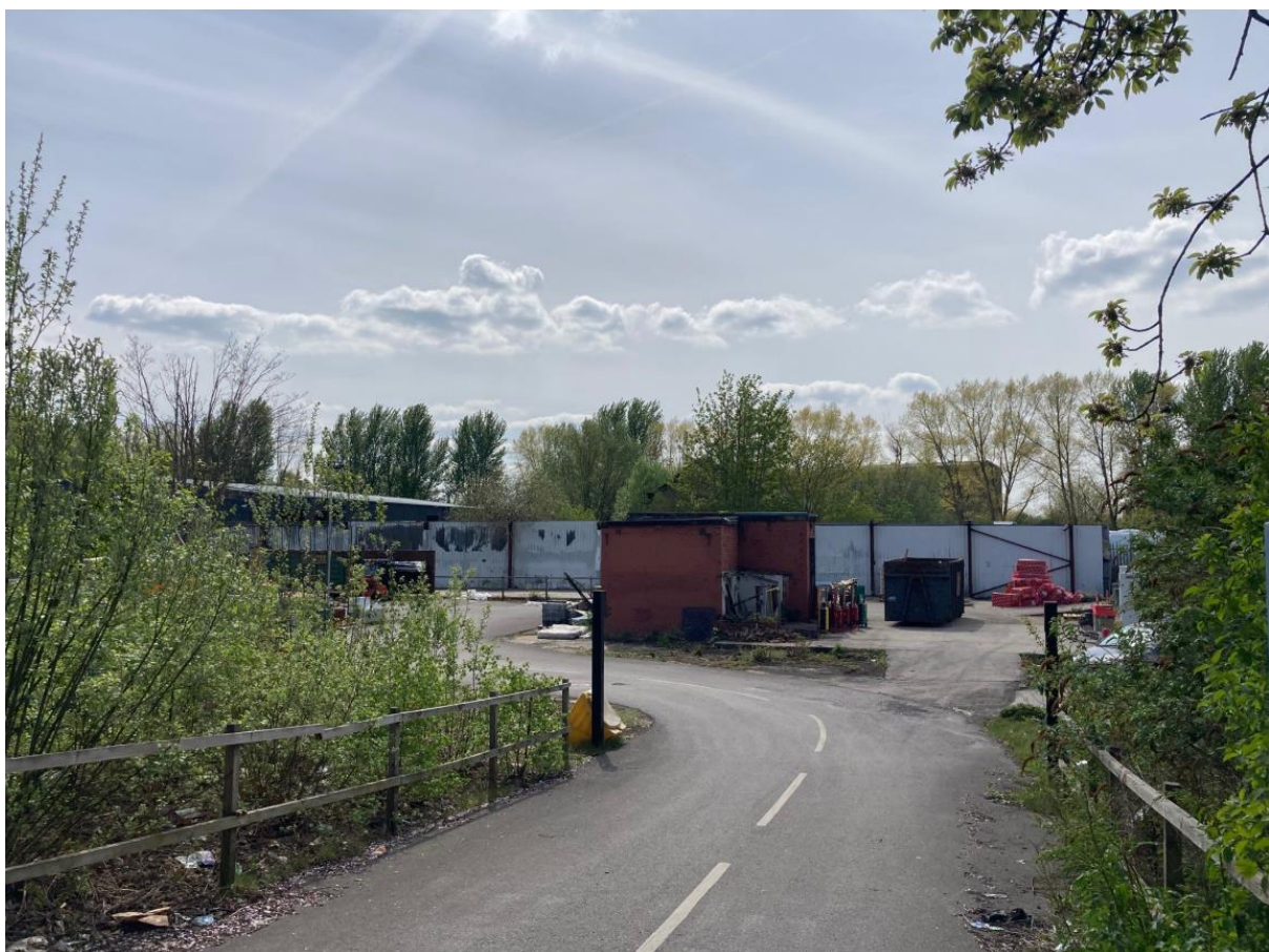
Photo 4: Site entrance from Globe Lane
